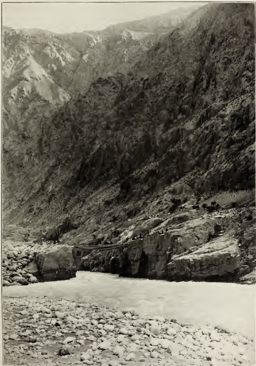
65. BRIDGE ACROSS YURUNG-KASH RIVER IN GORGE NEAR KHUSHLASH-LANGAR.
